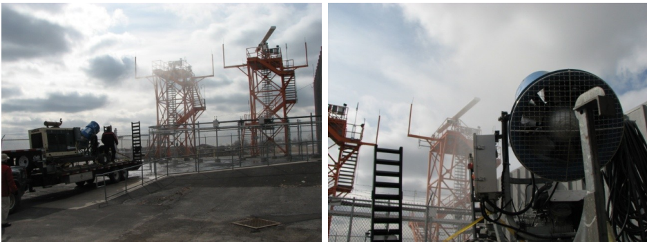
Figure 9. Blasting the EASAT Radome with Wet Snow and Ice
